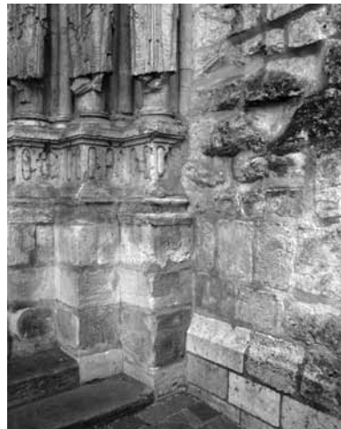
Etampes south portal, lower right
