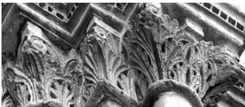
Saint-Denis W-wCR(cw) west window at the upper arrow in the elevation above 1137
