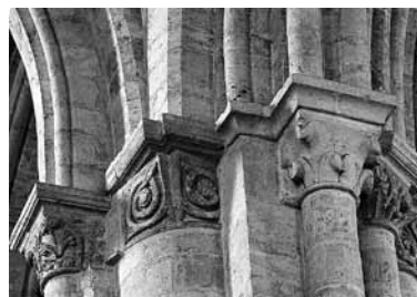
Etampes NE1 crossing pier, arrowed above
